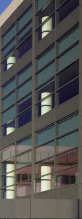
New building (at right in photo, facing page) frames an entrance forecourt. Glass skin (right) reveals the simplicity of structural frame.
